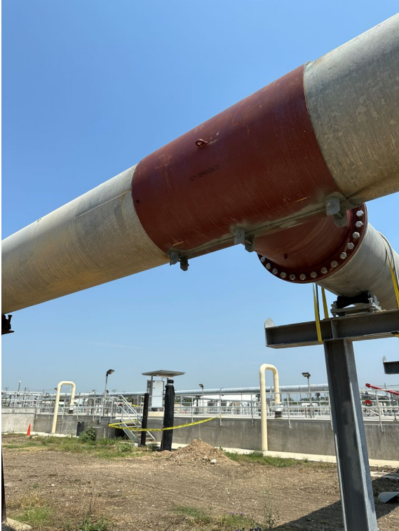
LPA Tie-in keeping 'new' and 'old'
