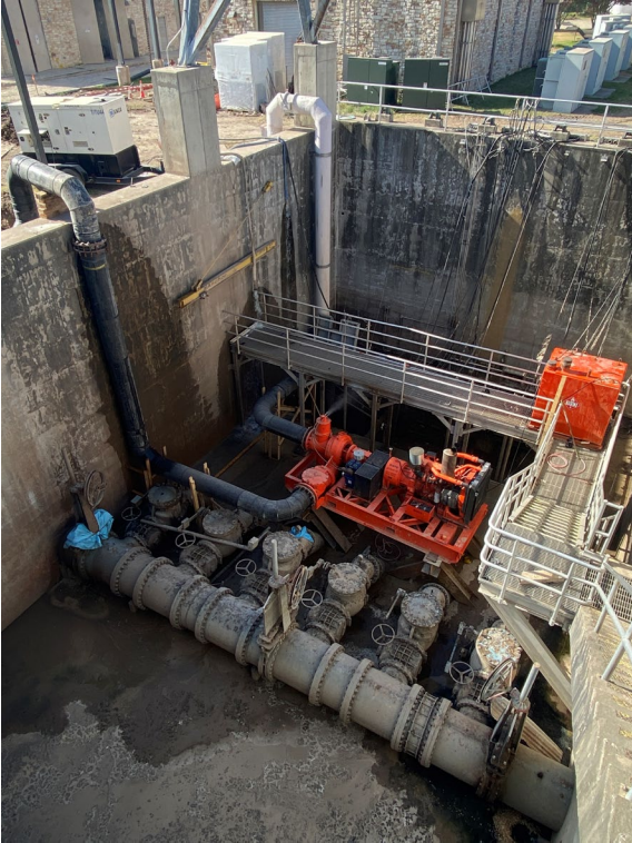
Tie-in new PTU (bypass pump)
