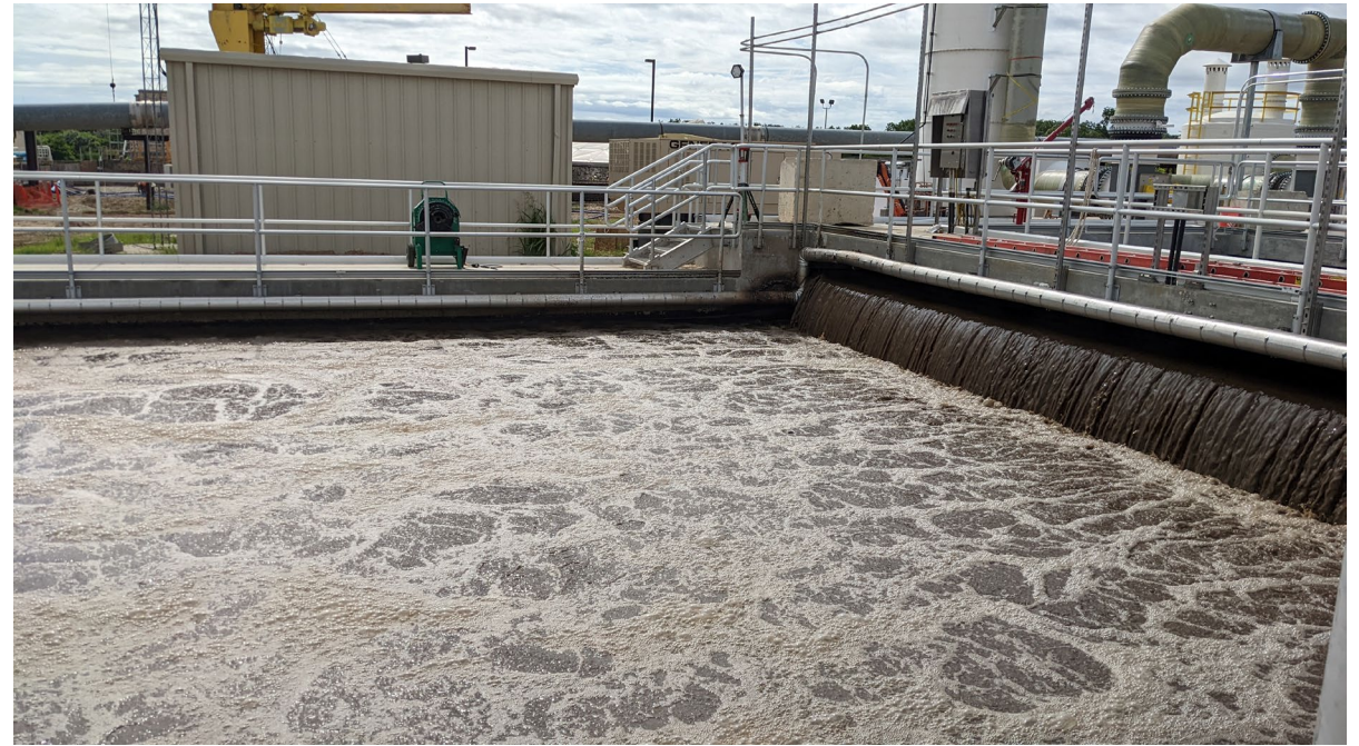
Train 3 flow from anoxic zone to aerated basin
