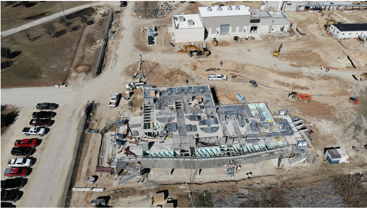
New 120 MGD Preliminary Treatment Unit Constructed
