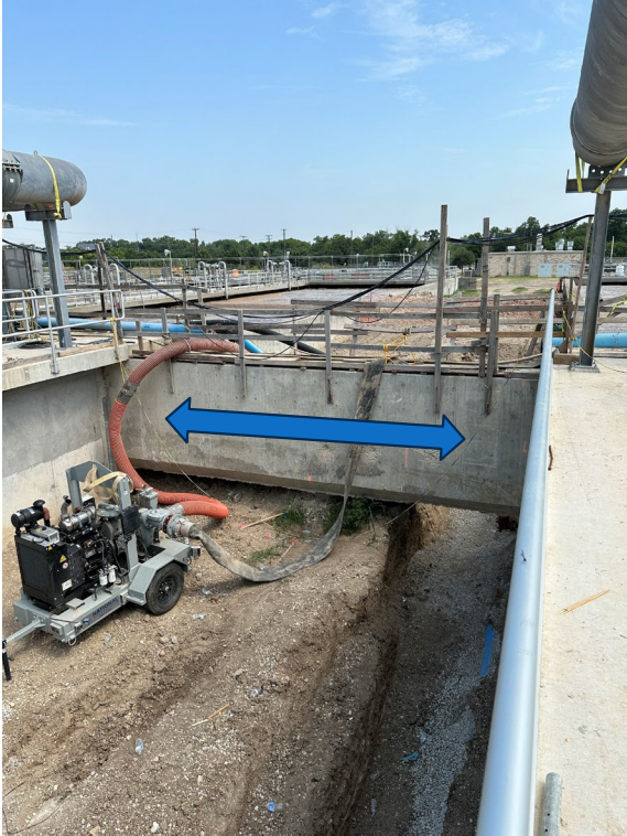
Temporary channel construction
