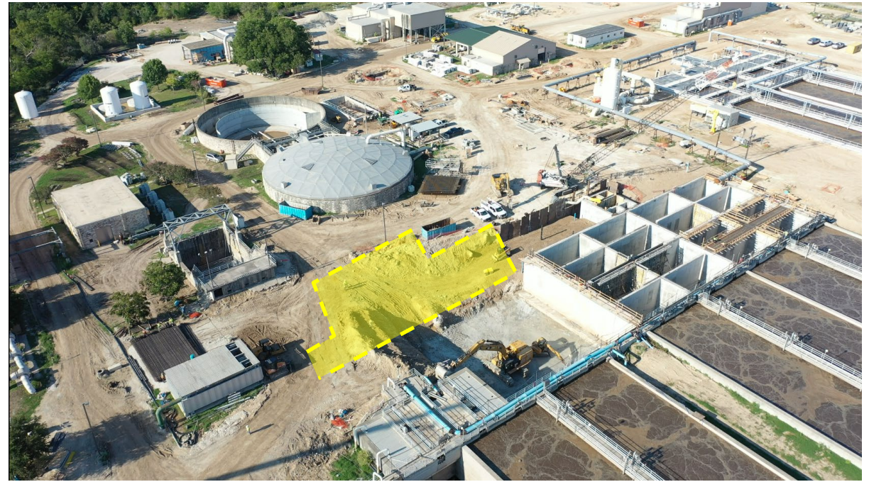
PTU removal and A&A zone construction
