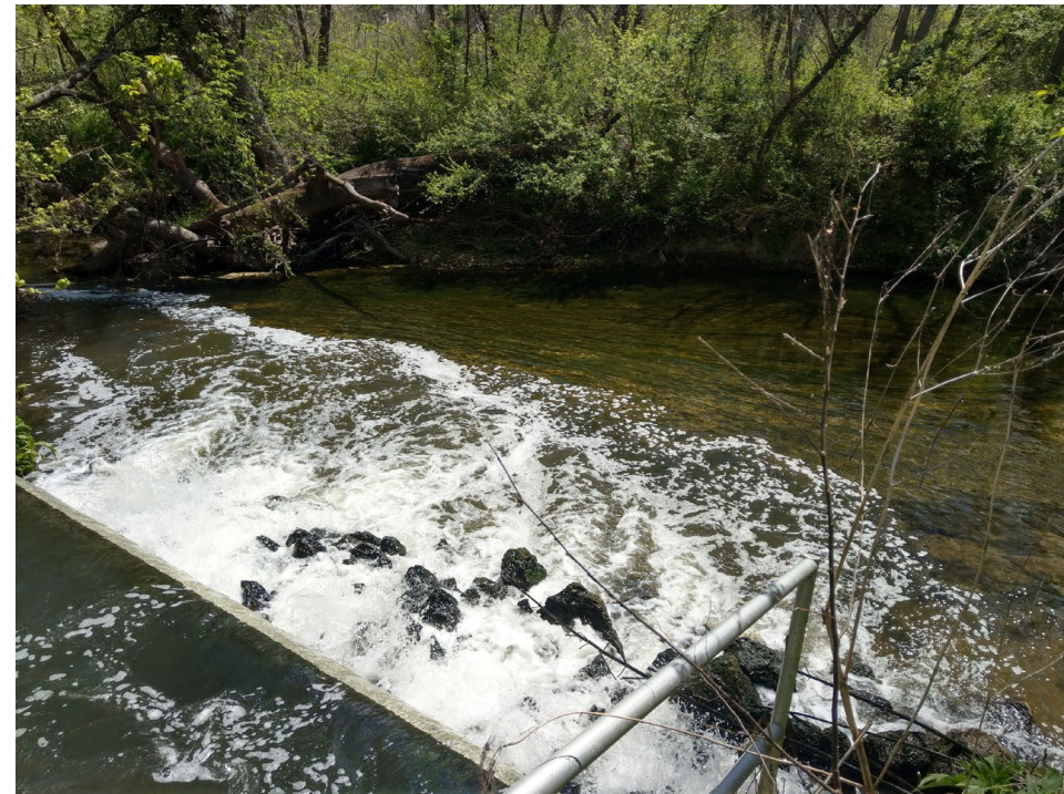
Outfall into Brushy Creek
