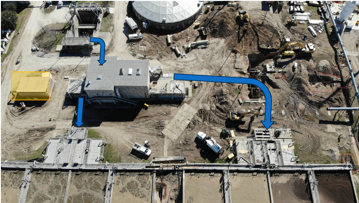
Existing Trains 1 & 2 Prior to major demolition
