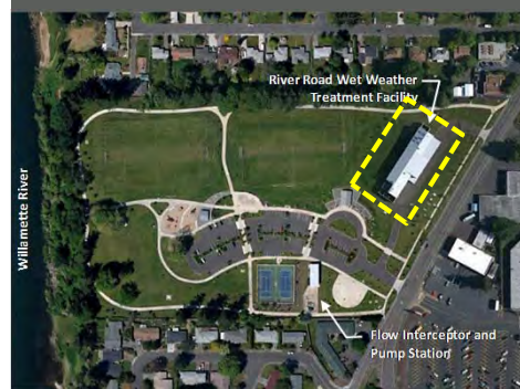
50-mgd River Road Park WWTF Salem, Oregon
