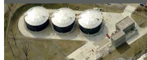
30-mgd SSO 700 Facility Cincinnati, Ohio
