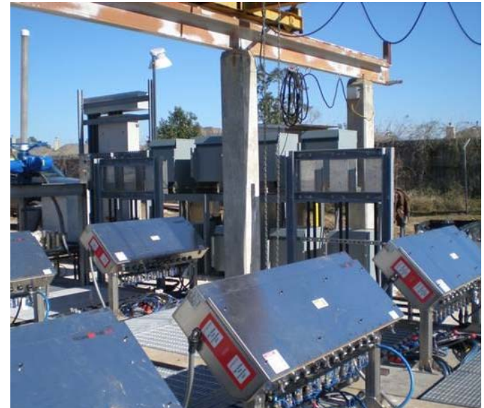
TROJAN UV AT BLACKHAWK WWTP
