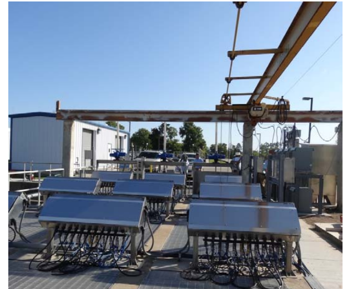
TROJAN UV AT BLACKHAWK WWTP
