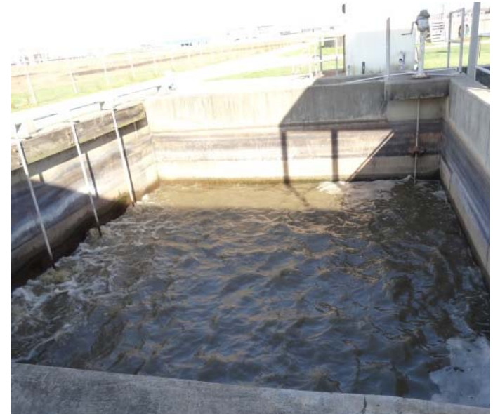
OLD CHLORINE CONTACT BASIN
