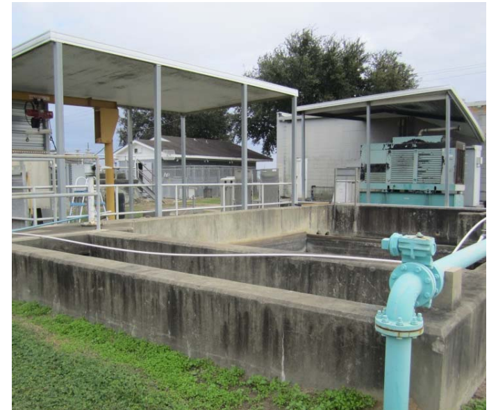
EXISTING UV AND CHLORINE CONTACT BASIN
