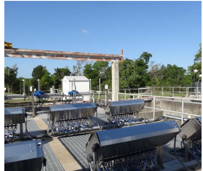
TROJAN UV AT BLACKHAWK WWTP
