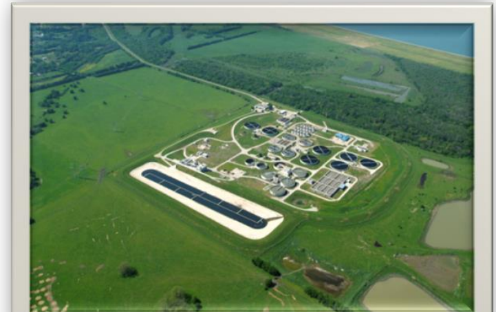
Duck Creek Treatment Plant
